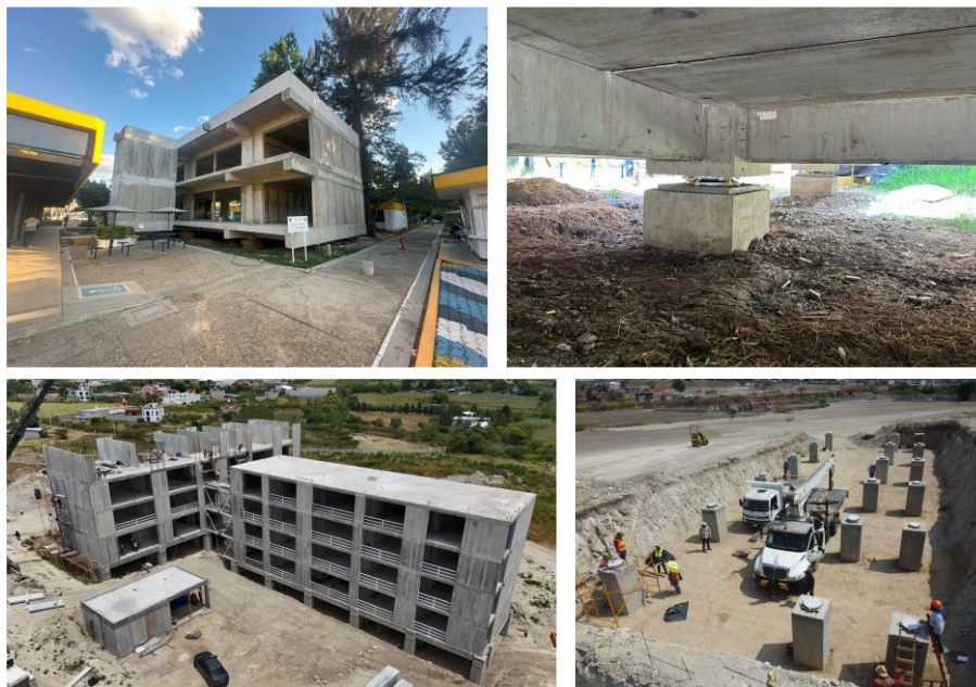
Figure 5. Educational facilities currently under construction in Oaxaca: a) Public, superstructure; b) Public, isolation system; c) Private, superstructure; d) Private, isolation system
